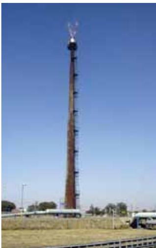
*The new enclosed ground flare at the Sasol Polymers ethylene plant in Sasolburg constructed to replace the open flare, the noise from which has been the subject of complaints by the nearby community.*
